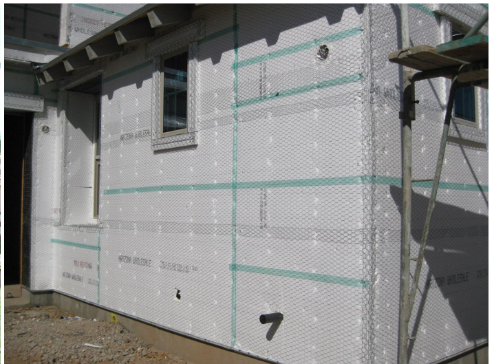
House 2. Sheathed with EPS board. Covered with Stucco Netting. Colored Stucco Next.
