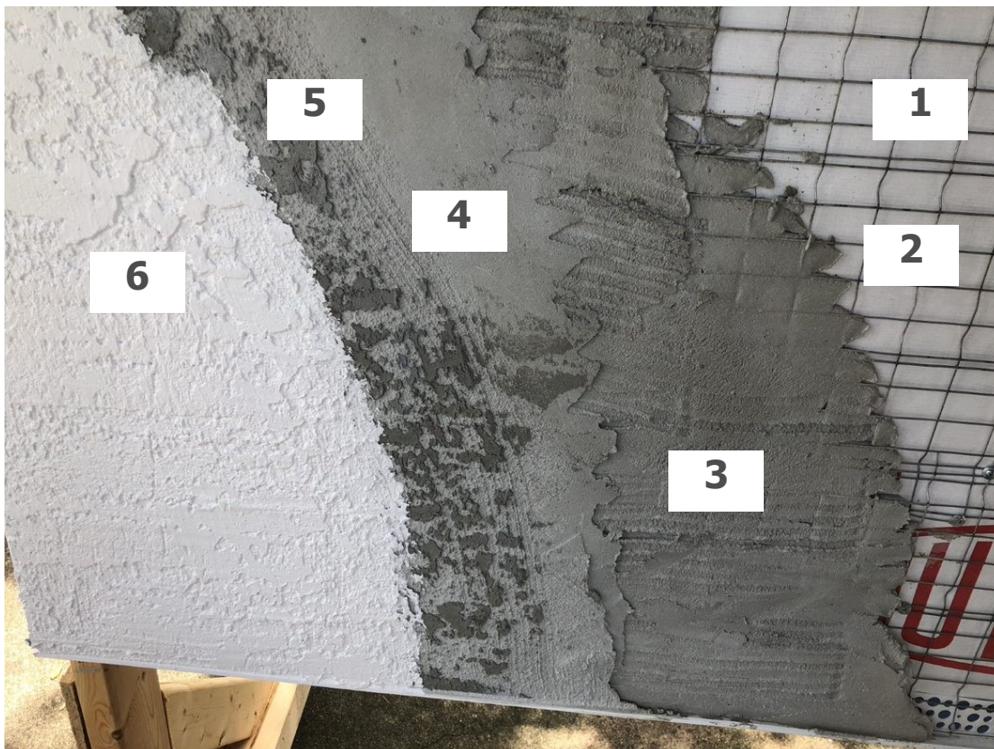
Figure 5 - Face Barrier Stucco System (Defined in ASTM 2128)
