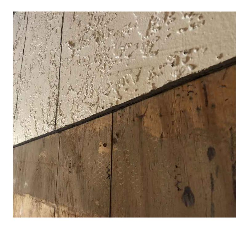
Un-Galvanized metal lath, no rust, no degradation, no water stains, no moisture deterioration. Just like the day it was put on 35 years ago.
