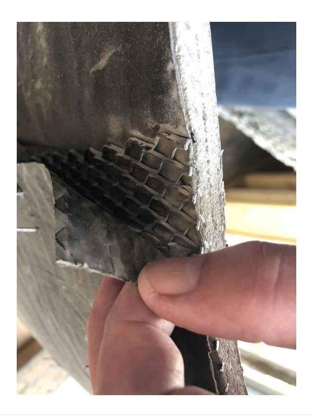
No Weep Screed—Lath brought over block and stub-nailed. Un-Galvanized metal lath, no rust, no degradation, no water stains, no moisture deterioration. Just like the day it was put on 35 years ago. Constant weather exposure in Florida's environment. No wood degradation whatsoever.
