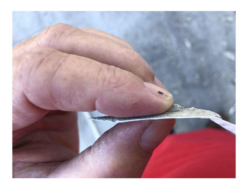
Back side of metal lath on the wall - Un-Galvanized metal lath, no rust, no degradation, no water stains, no moisture deterioration. Just like the day it was put on 35 years ago. Constant weather exposure in Florida's environment. Lap paper over metal. Still no Cracks, No faults, No flaws. Note staple attachment.
