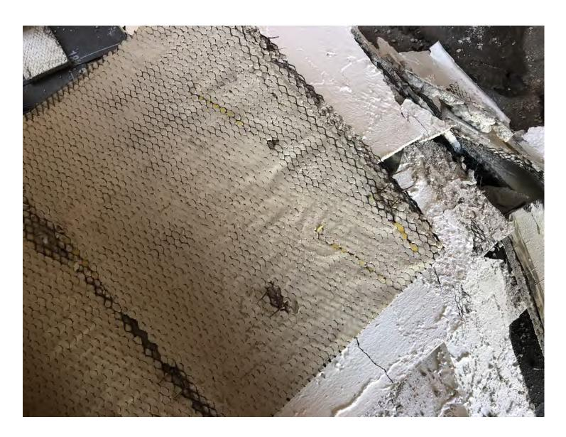
Un-Galvanized metal lath, no rust, no degradation, no water stains, no moisture deterioration. Just like the day it was put on 35 years ago. Constant weather exposure in Florida's environment. Lap paper over metal. Still no Cracks, No faults, No flaws. Photo from back side of removed panel.
