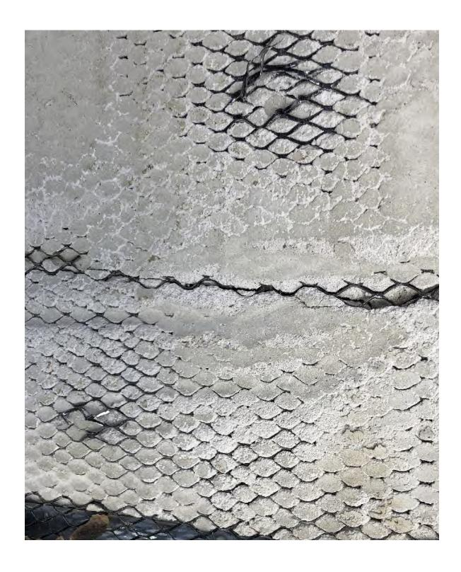
Un-Galvanized metal lath, no rust, no degradation, no water stains, no moisture deterioration. Just like the day it was put on 35 years ago. Lath shiny where cut through.
