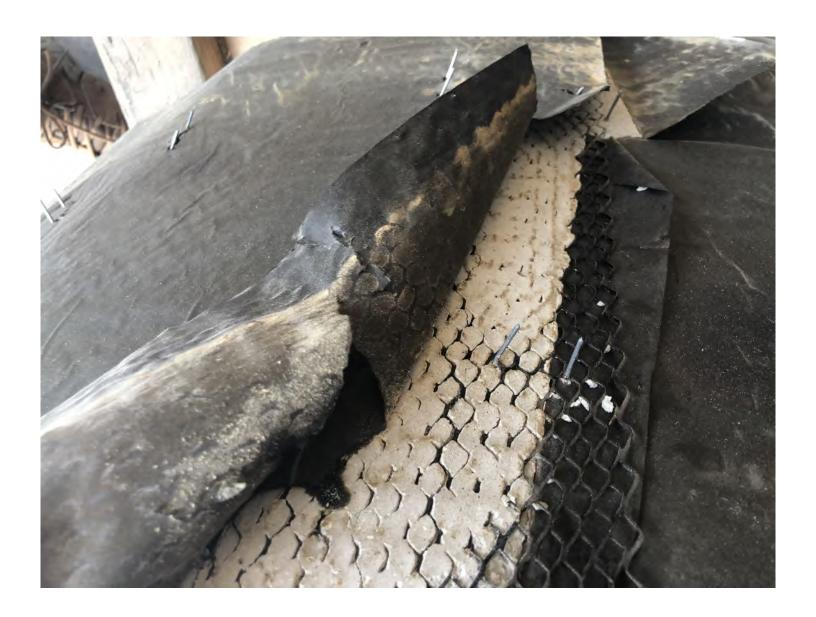
Back side of 1/2" exterior expanded flange casing stop used at bottom of stucco fascia. No weep, nor drainage, 35 years exposed to the weather, looks like the day it was installed. No leaks, No faults, No flaws, No cracks, No rust.
