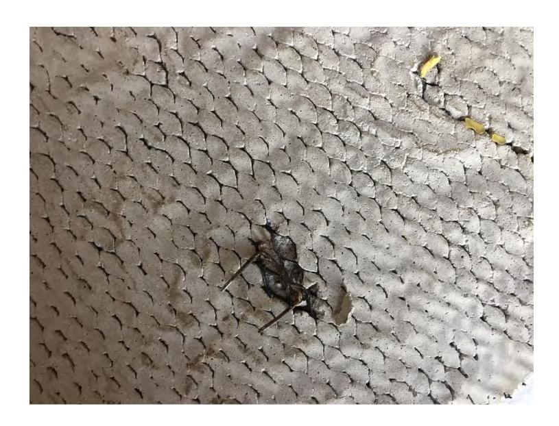
Paper over lath & back lap - No cracks, No leaks and No faults.
