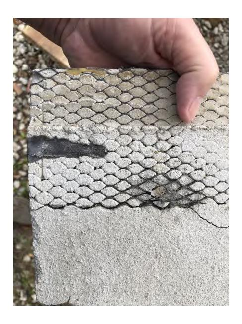
No Weep Screed—Lath brought over block and stub-nailed. Un-Galvanized metal lath, no rust, no degradation, no water stains, no moisture deterioration. Just like the day it was put on 35 years ago. Constant weather exposure in Florida's environment. No wood degradation whatsoever on sheathing.
