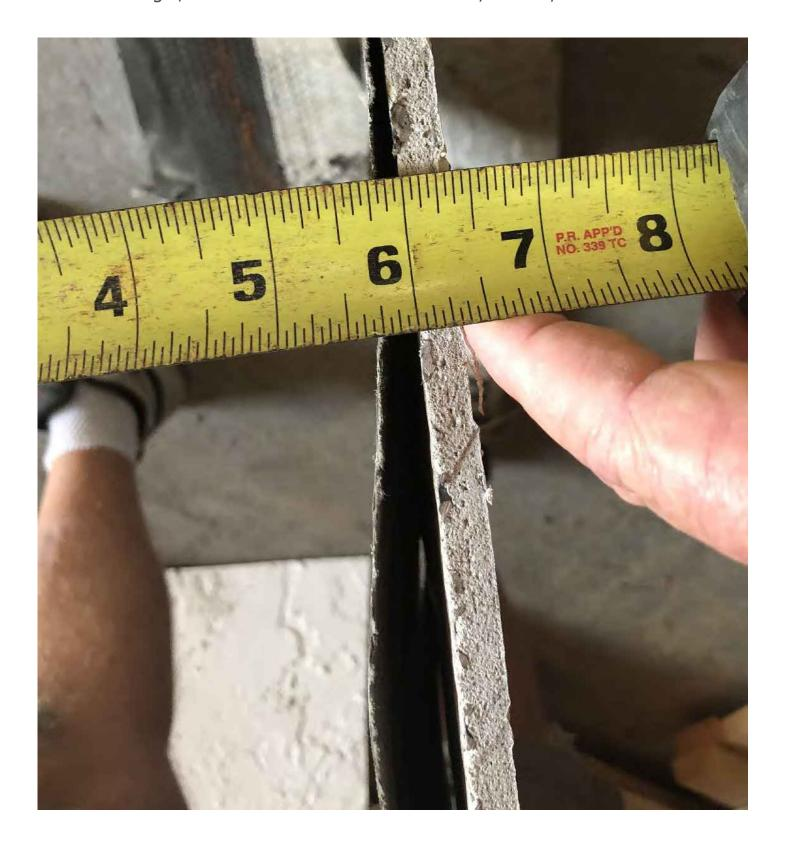
Un-Galvanized metal lath, no rust, no degradation, no water stains, no moisture deterioration. Just like the day it was put on 35 years ago.
