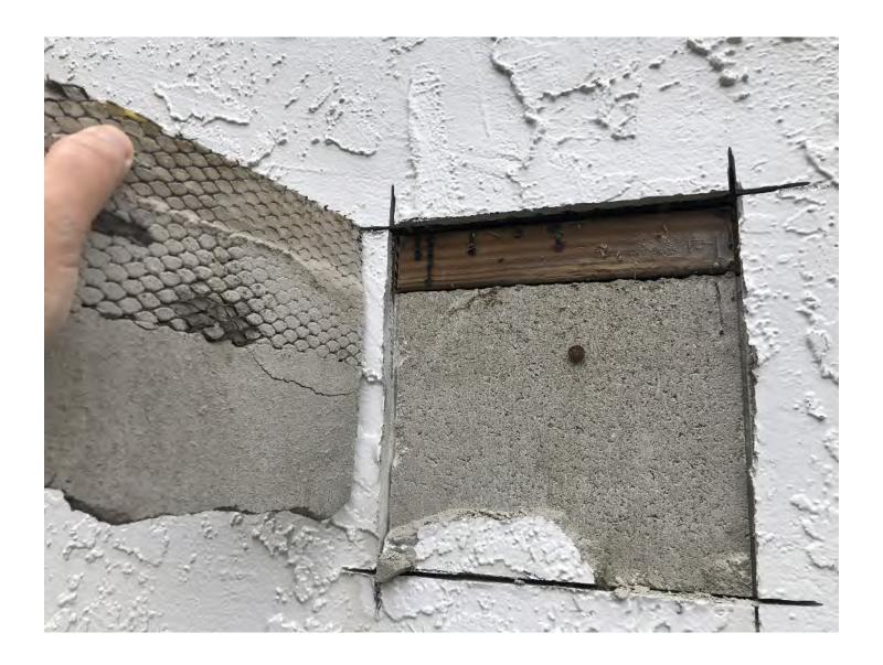
35 year old frame to block wall transition. Un-Galvanized metal lath, no rust, no degradation, no water stains, no moisture deterioration. Just like the day it was put on 35 years ago. Constant weather exposure in Florida's environment. Lap paper over metal. Still no Cracks, No faults, No flaws, and No weed screed.
