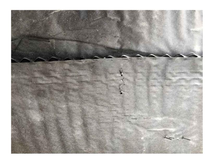
Un-Galvanized metal lath, no rust, no degradation, no water stains, no moisture deterioration. Just like the day it was put on 35 years ago. Constant weather exposure in Florida's environment. Note paper over lath - No cracks, No faults, No flaws.
