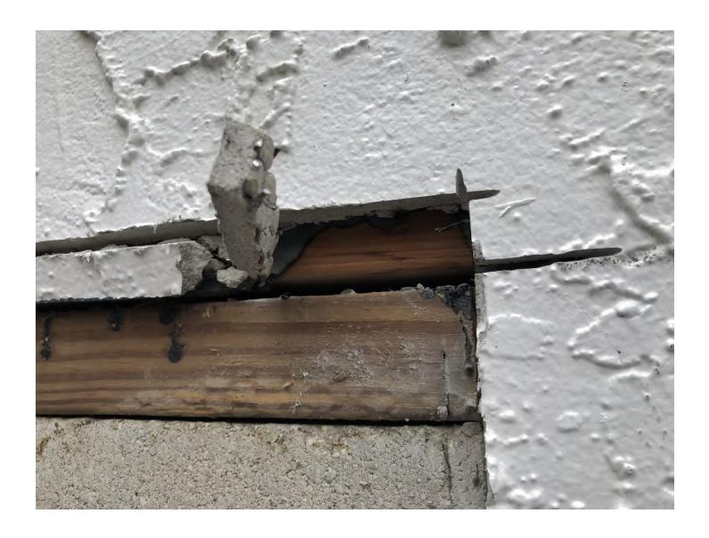
Stucco Cladding 1/2" Nominal Thickness - applied using South Florida Building Code requirement or using the ASTM "unless specified otherwise" provision. No cracks anywhere.
