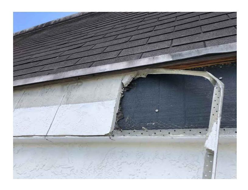
Upper section of rear wall with Stucco Fascia removed ready for back wall scoring.
