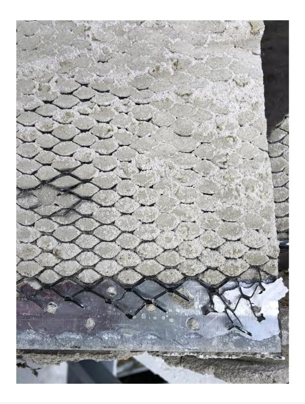
Back side of 1/2" exterior expanded flange casing stop used at bottom of stucco fascia. No weep, nor drainage, 35 years exposed to the weather, looks like the day it was installed. No leaks, No faults, No flaws, No cracks, No rust.
