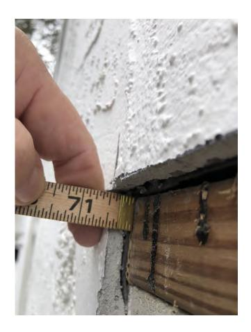
Stucco interface with window separated by Sealant. No casing separating the frame, no backer rod, just a "V" groove and sealant. Always has worked flawlessly. Always will if done properly.
