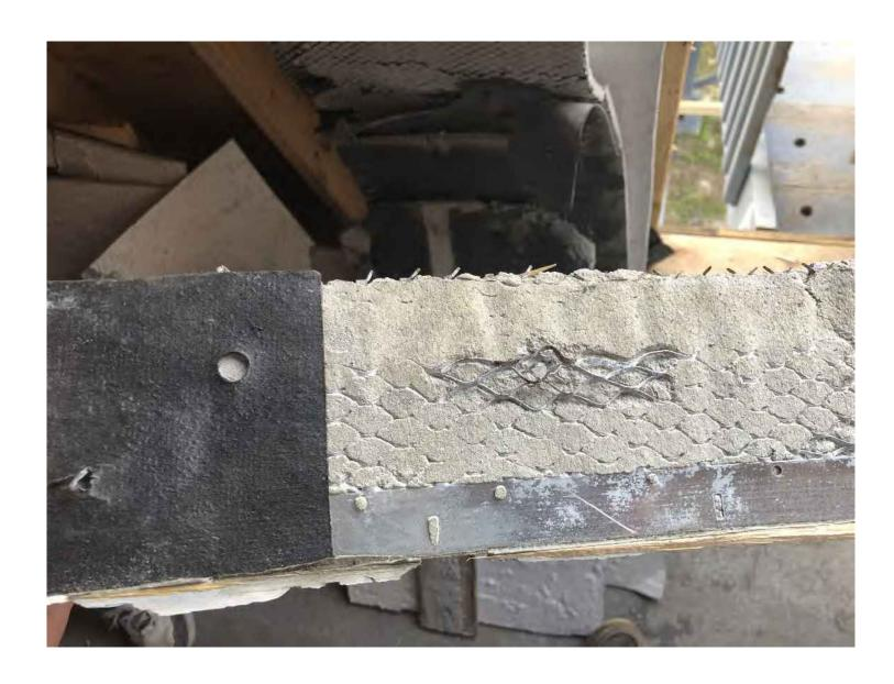
Stucco Cladding painted twice in 35 years, original paint and white re-paint. Both followed standard painting instructions and was applied with rollers to the standard mill thickness required for exterior cement plaster installation.
