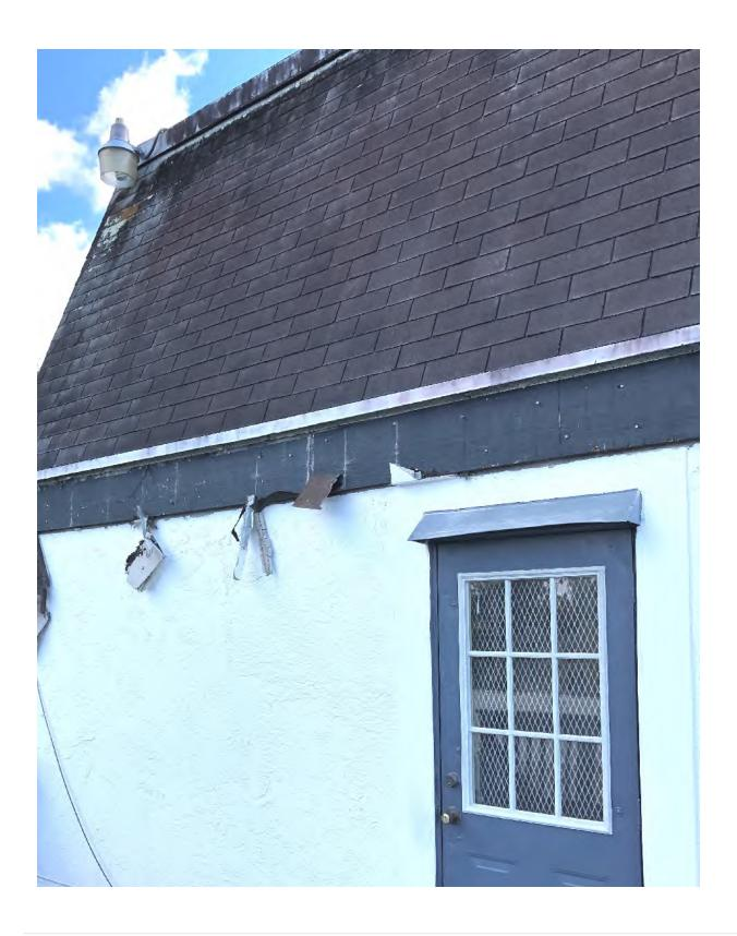
Rear Wall with scoring to remove stucco assembly. Stucco Cladding had zero cracks, zero leaks, zero faults. We will later look at the back side of the lath.
