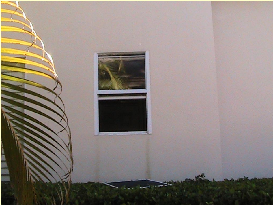
Photo W-6 – Flush window installation – No casing separation
