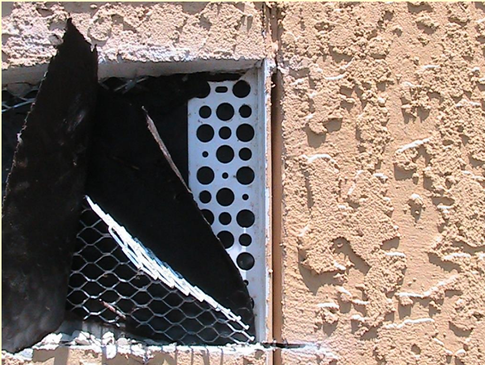
Paper over flange provides a direct water route to substrate
