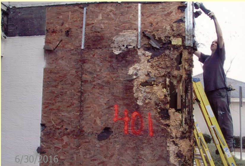
Photo C-3 – Where the Plastic corner bead was improperly installed, sealed and prepped for stucco.
