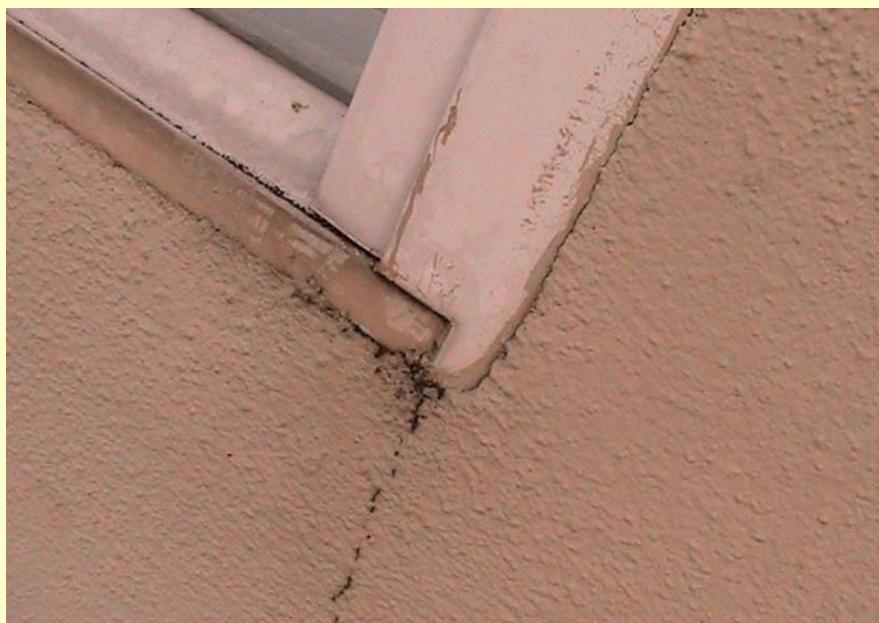
Photo W-14 – Close up – Window jamb/sill leak. Although as previously stated, the remediation protocol will seal the perimeter frame also.
