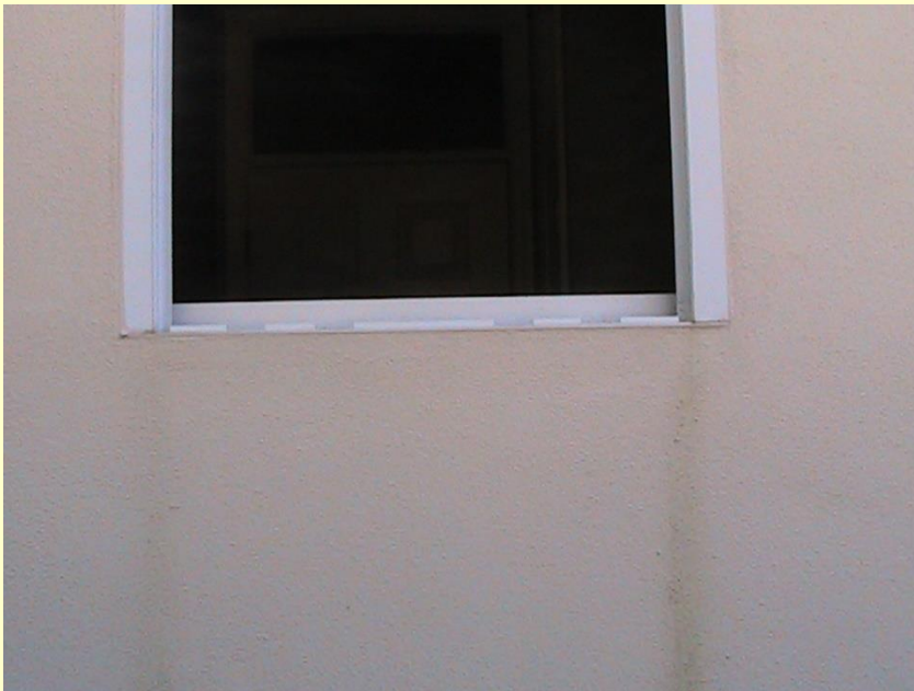
Photo W-6 – Flush window installation – No casing separation
