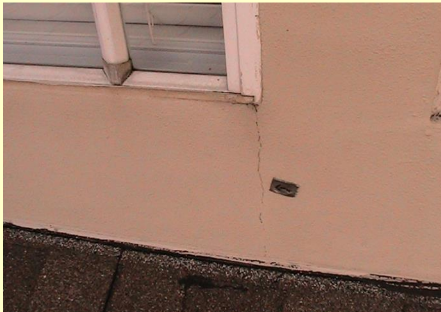
Photo W-14 – Close up – Window jamb/sill leak. Although as previously stated, the remediation protocol will seal the perimeter frame also.
