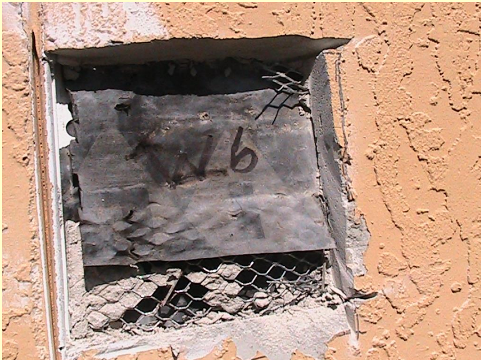
Paper over flange provides a direct water route to substrate
