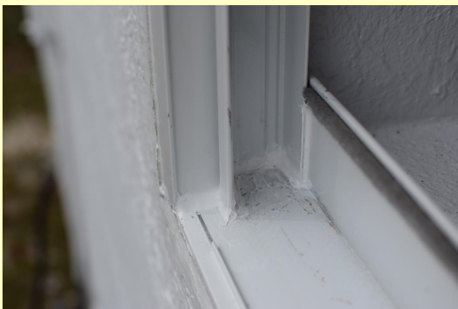
Photo W-11 – Example window jamb/sill joint repair
