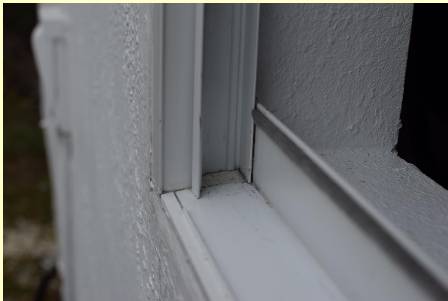
Photo W-10 – Example window jamb/sill joint leak
