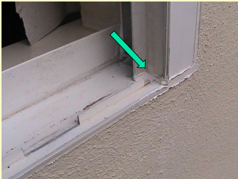
Photo W-9 – Close up – Perimeter separation repair complete
