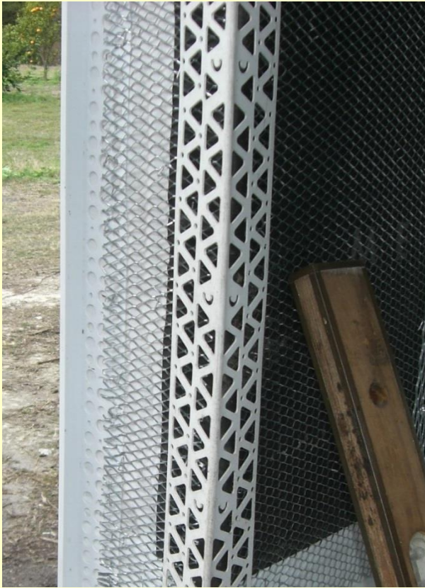
Photo C-3 – Where the Plastic corner bead was improperly installed, sealed and prepped for stucco.
