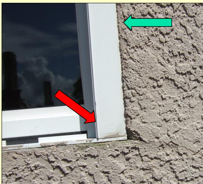
Photo W-4 – Close up of window with flush wall stucco
